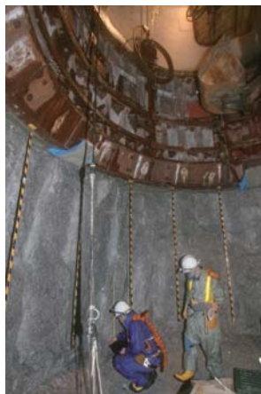
換気立坑 (深度490.4m)
